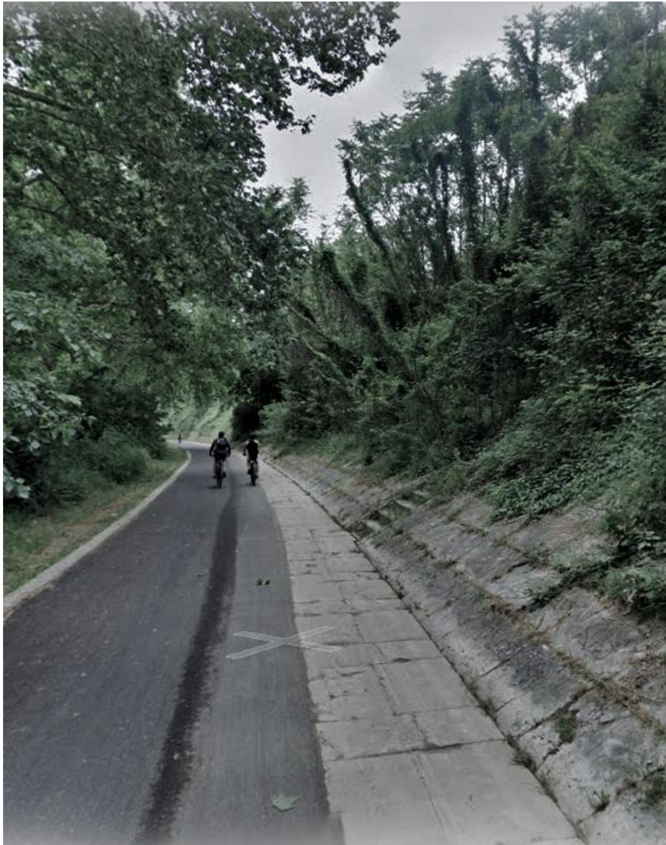
Before: River Walkway
